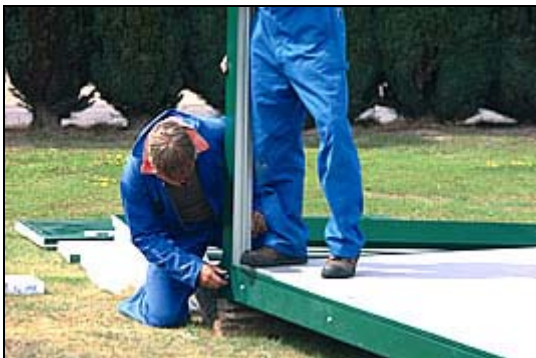
Fix the four corner posts
