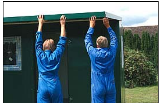
Fit the outer roof skin
