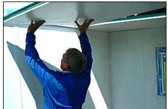
Slide in the ceiling panels
