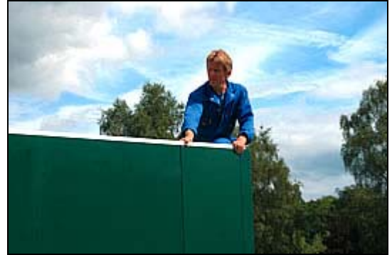
Fit the ceiling retention bars
