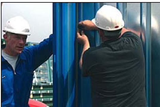
Fix the holding screws
