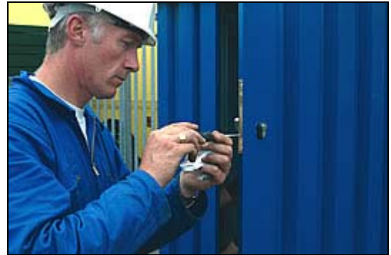
Install the two door locks
