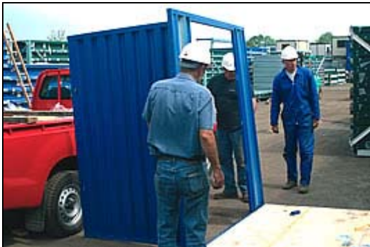
Fit panels to the Expandastore base
