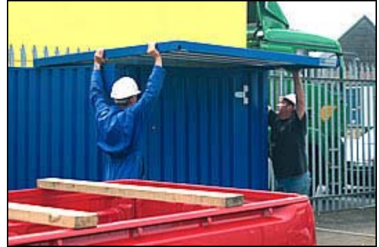
Lift on & fix the roof
